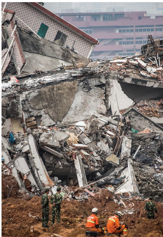
Construction waste collapse in Shenzhen, China.
